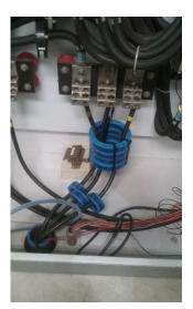
**Reality:** CoolBlue inductive absorbers do not affect symmetrical power currents. They do suppress asymmetrical radio frequency noise currents as well as asymmetrical electromagnetic interference (EMI) currents that are generated by the parasitic capacitances of the system itself, including the motor cable. This efficient dampening of destructive asymmetrical currents creates a common mode choke.
